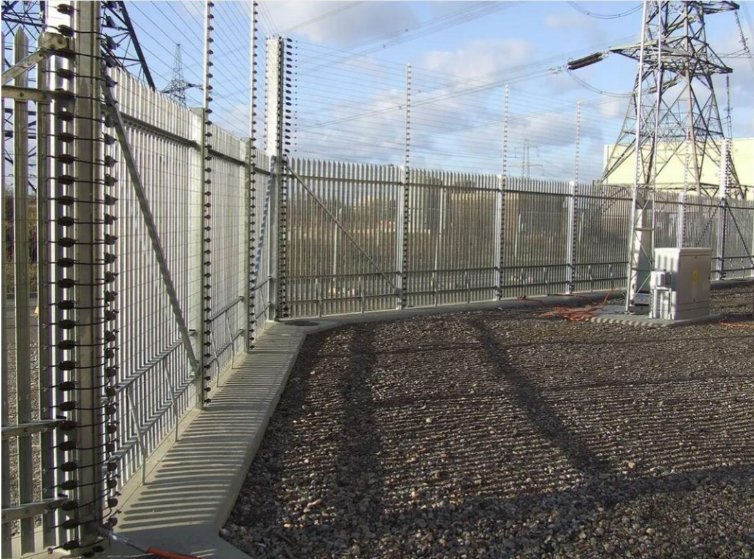
Plate 4.5 Typical examples of high security external fencing
